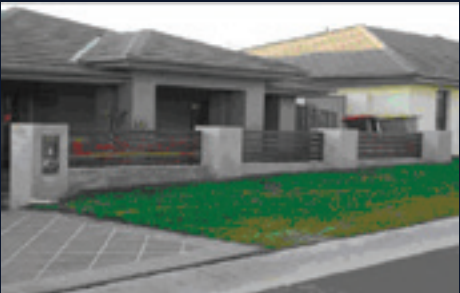
Figure 2.15. Front fencing with infill panels
