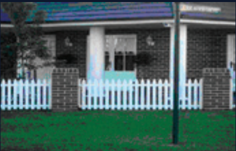
Figure 2.16. Face brick piers with picket
